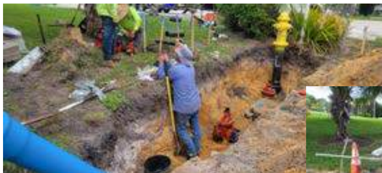
Above: The installing of the new water main and fire hydrant. To the right is an update of the work at the ending of September.
