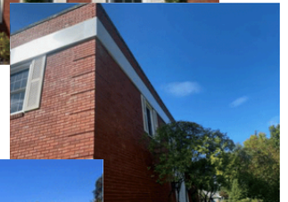
Replaced exterior fascia
