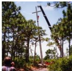
Cross Tower going up
