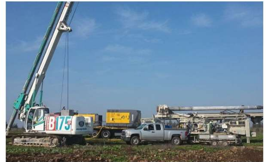
Heavy machinery for exploratory oil drilling on the Golan Heights at Oil Site 5. (Courtesy Afek Oil and Gas)
