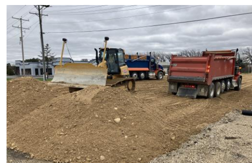
Granular sub-base being spread
