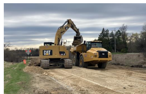
Existing asphalt being removed
