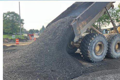
Aggregate base course (recycled pavement) being offloaded
