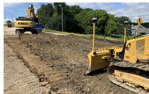
Excavation of existing subgrade materials
