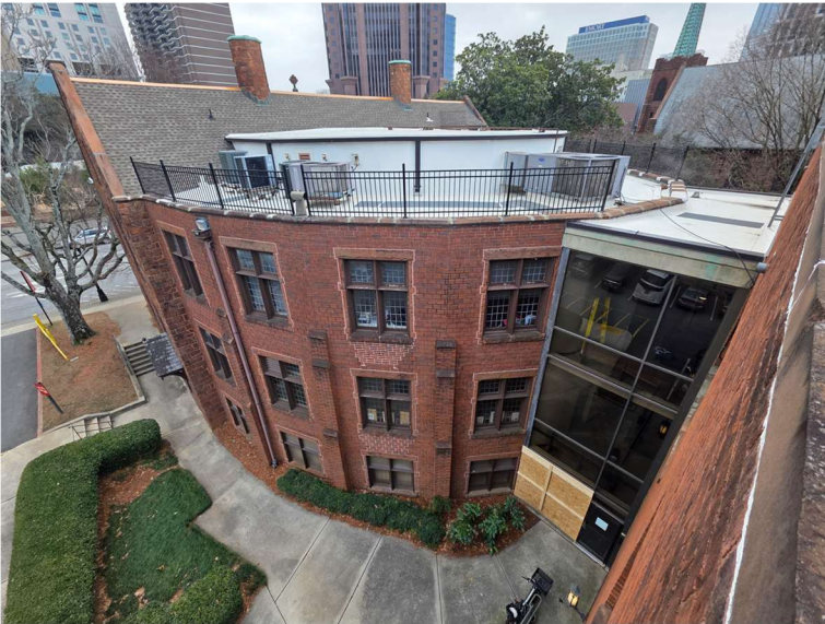
Photo 6: View of north façade of Egleston.
