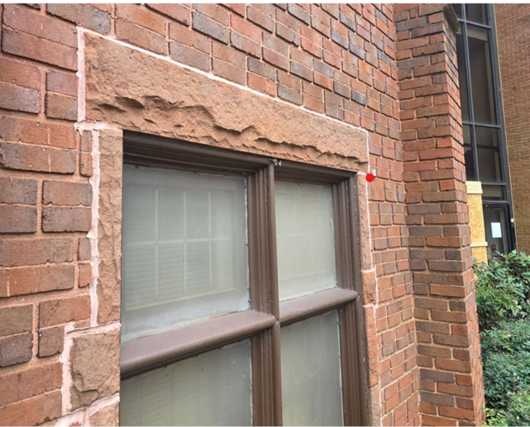
Photo 38: Egleston window with polycarbonate storm window atop wood window sash.
