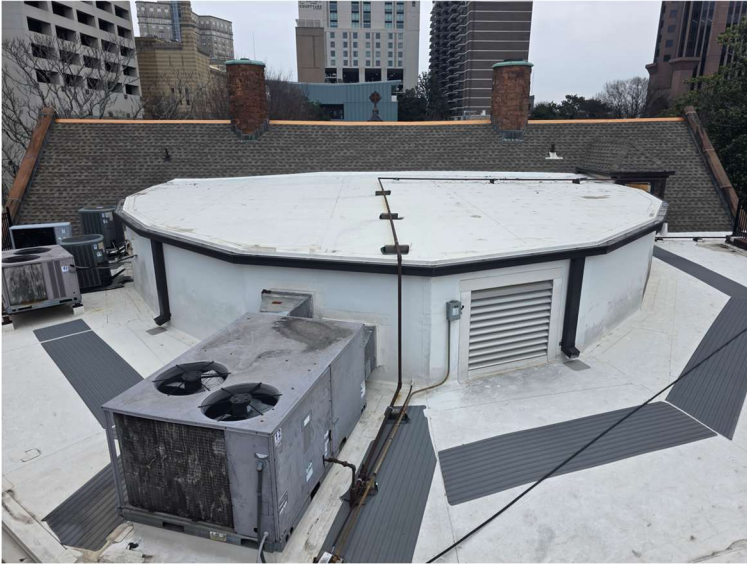
Photo 7: Overall view of Egleston roofs.
