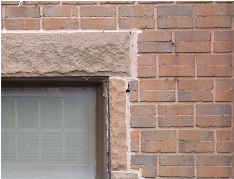
Photo 30: Egleston sealant repair at jamb stone quoins with joint gaps.
