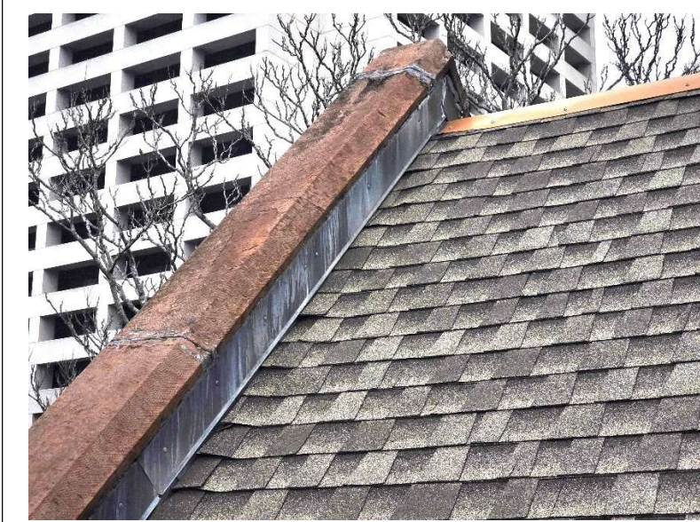
Photo 13: View of Egleston asphaltic shingle roofing.
