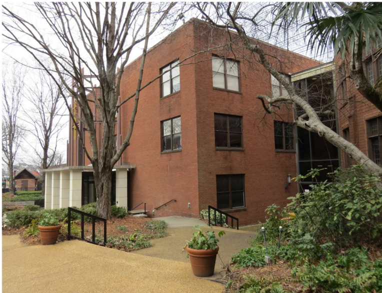
Photo 4: Overall view of Parish House, south elevation.
