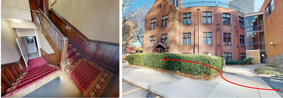
FIGURE 5 THE ACCESSIBLE ROUTE FROM ADA PARKING IS BLOCKED BY STAIRS ONCE INSIDE THE BUILDING
