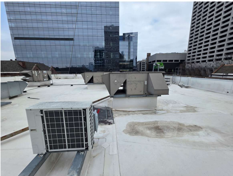
Photo 8: Overall view of Parish Hall roof.
