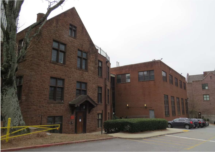
Photo 1: View of Egleston (left) and Parish House (right).
