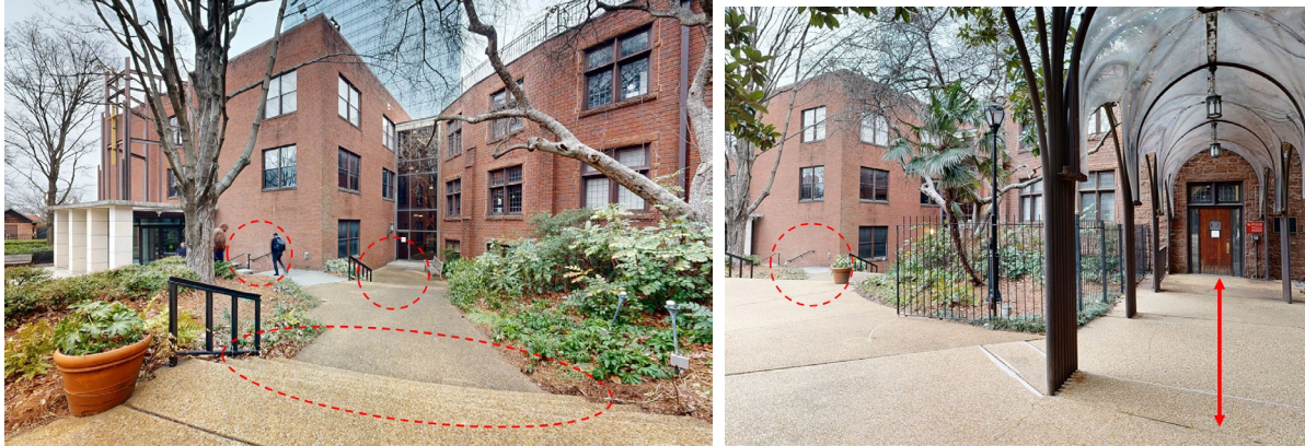
FIGURE 3 EXTERIOR STAIRS LIMIT ACCESSIBILITY INTO EGGLESTON HALL FROM THE COURTYARD
