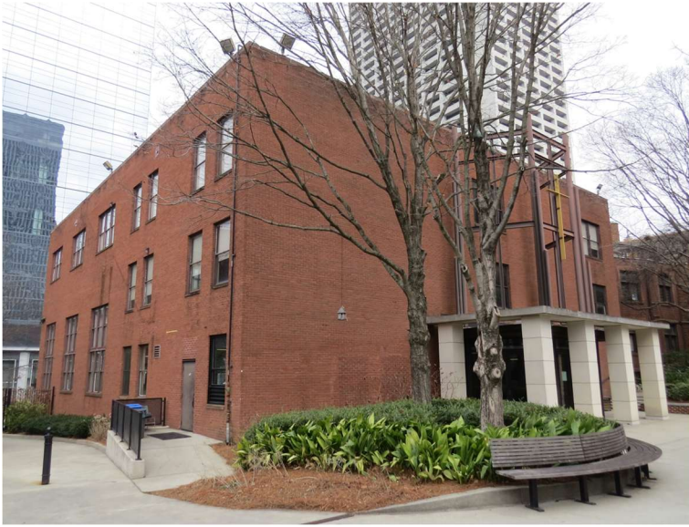
Photo 5: Overall view of Parish House.
