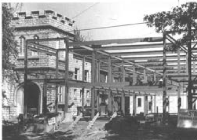
A steel skeleton outlines the new educational building under construction.
