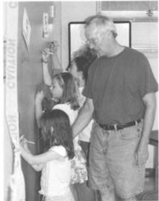
Right: Children write on soon-to-be demolished walls during celebrations marking the start of Fellowship Hall renovations in 2005.
