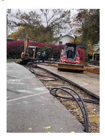
At the end of the trenches, a large hole is being dug to allow for these tubes to pass underneath the brick alley, into the current boiler room. Once the hole is excavated pipes will be pushed beneath the alleyway, hopefully without having to disturb any of the bricks.
