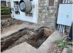
Last week excavation on the new mechanical room beneath the choir loft began taking shape, as dirt is being removed by the 5-gallon bucket full and the wheelbarrow full. The black poles in the picture are temporary supports that will be removed once steel reinforcement is added to the ceiling of the space.
