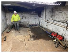
Beneath the sanctuary, trench work is well underway to make space around the sanctuary's perimeter for new ductwork. As of this writing the trench has reached from the organ console to the back corner of the sanctuary (organ side). Because all that dirt must be dug by hand, a conveyer system was added to move the dirt from the far reaches beneath the sanctuary back to the new mechanical room, where it can be wheelbarrowed out of the building. (pictured on the left below)
