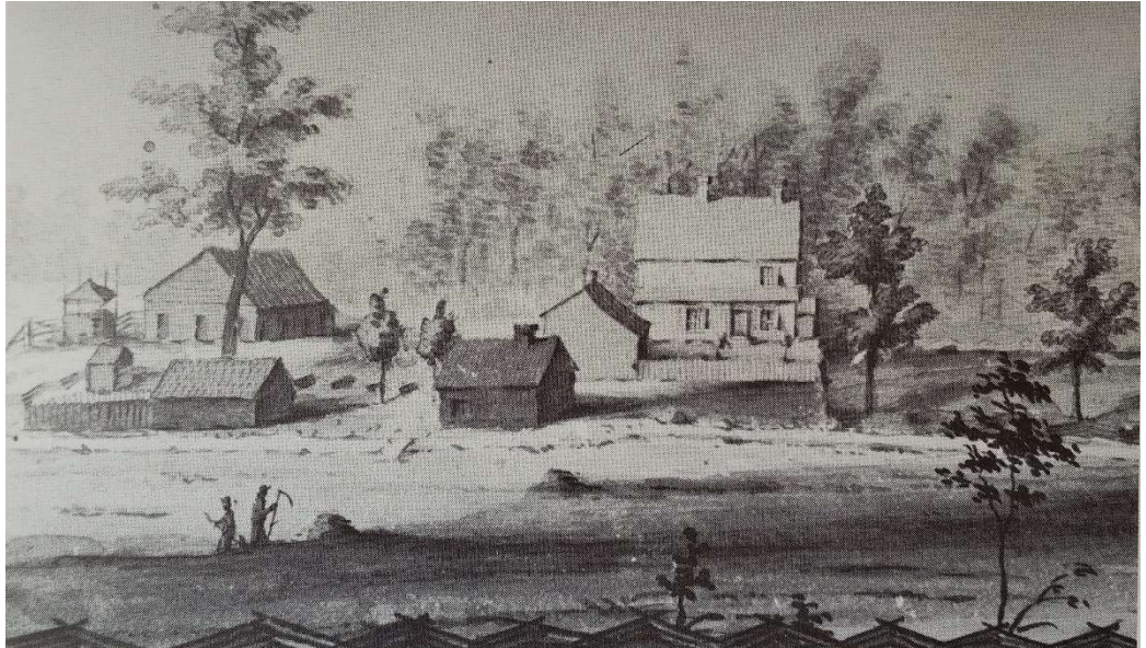
The Pilgerhaus (Pilgrim's House) Built by John George Klein to house itinerant ministers 1757 Drawing by Nicholas Garrison, Jr.
